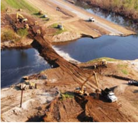
Levee reconstruction - New Orleans, LA
