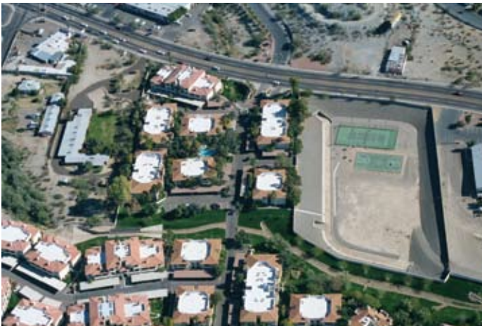
Multi-use Urban Retention Basin - Phoenix, AZ
