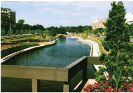
Flood Protection - Kansas City, KS
