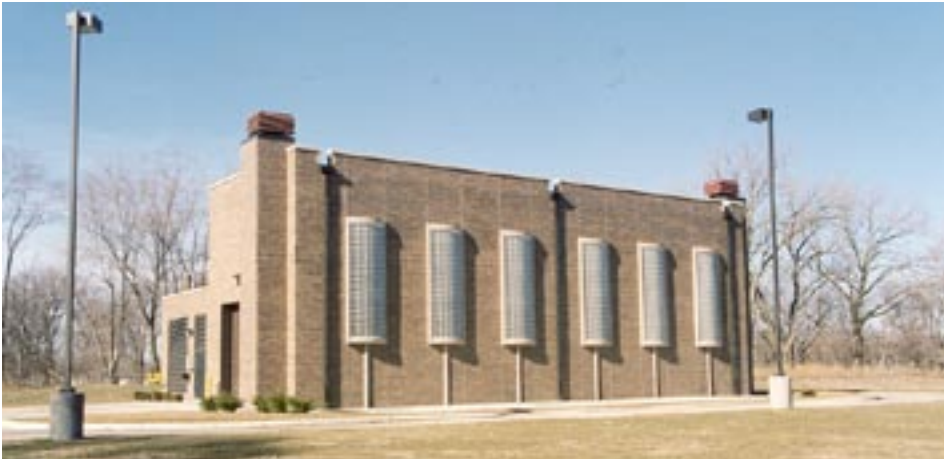
Pump Station Upgrade
