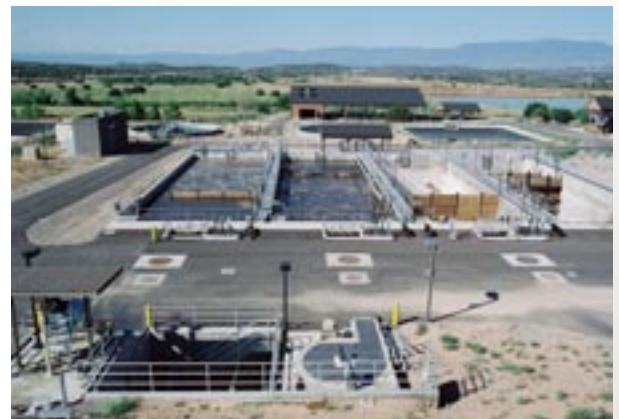
Treatment Plant Upgrade
