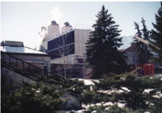
Cooling Tower Replacement
