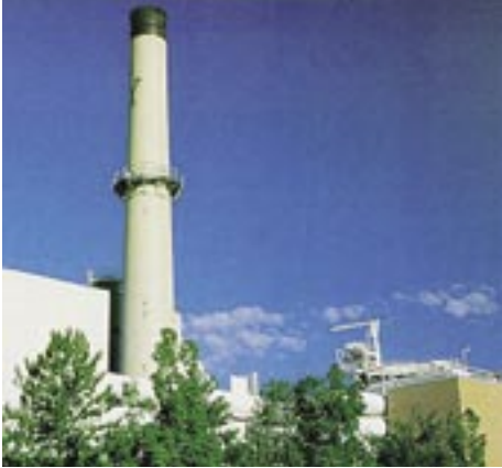
Central Heating Plant
