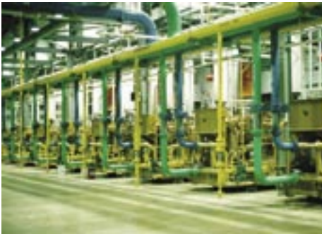
Stand-by Generation Facility
