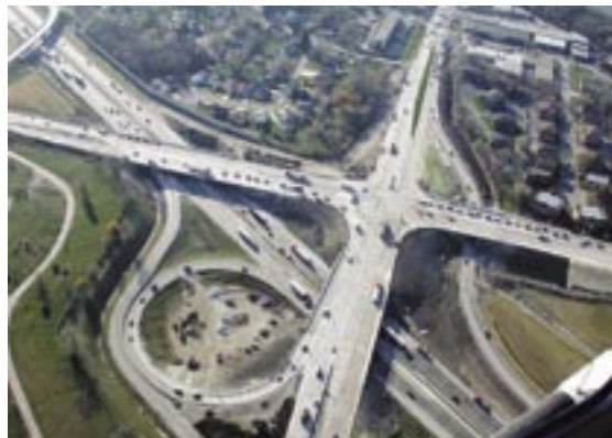
Reconstruction and Widening
